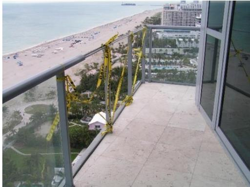
Figure 1: Damaged GHRs from hurricane Wilma
