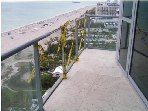
Figure 1: Damaged GHRs from hurricane Wilma
