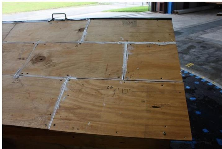
Figure 47. Unsealed gap between sheathing
